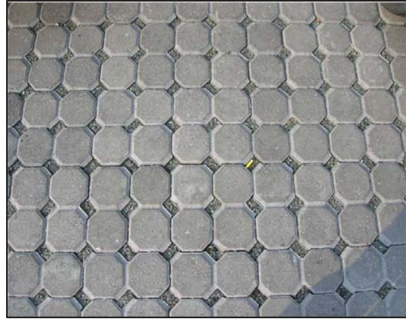
Permeable/Porous Pavement (Photograph courtesy of VADEQ)
