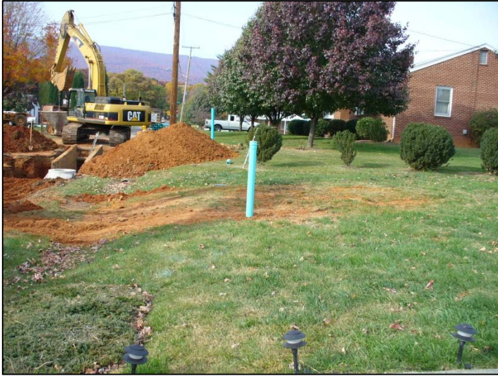
Western VA Water Authority Sewerline Connection (Photograph courtesy of WVWA)
